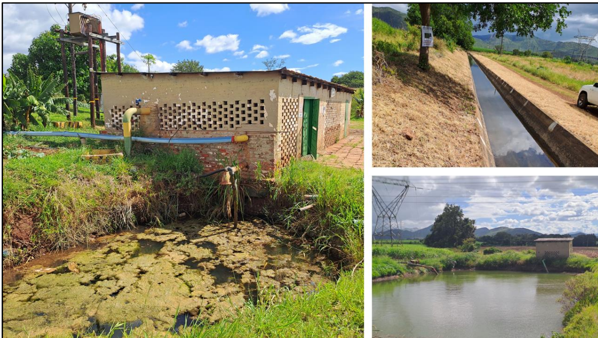
Figure 13: Water impoundment areas.
